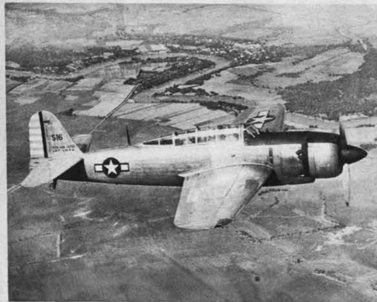
Radial Judy has low mid-wing unusual in Jap planes. As on other Jap light bombers, greenhouse is long and high. Fuselage appears clean.
